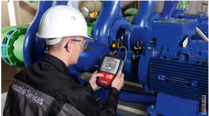
Figure 7 Shaft alignment device FAG Top-Laser EQUILIGN
